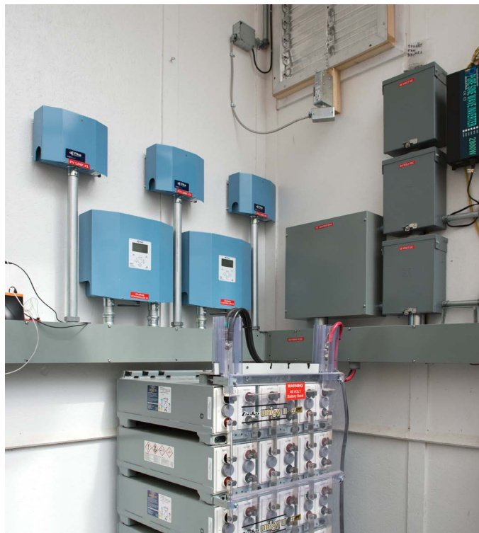
Charge controllers and batteries in the bioshelter
