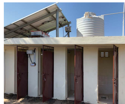
Bank of toilets with solar pump for running water
